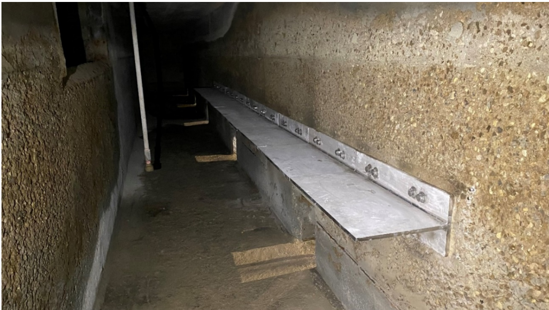
Figure 5: New baffle wall installed in flocculation tank.
