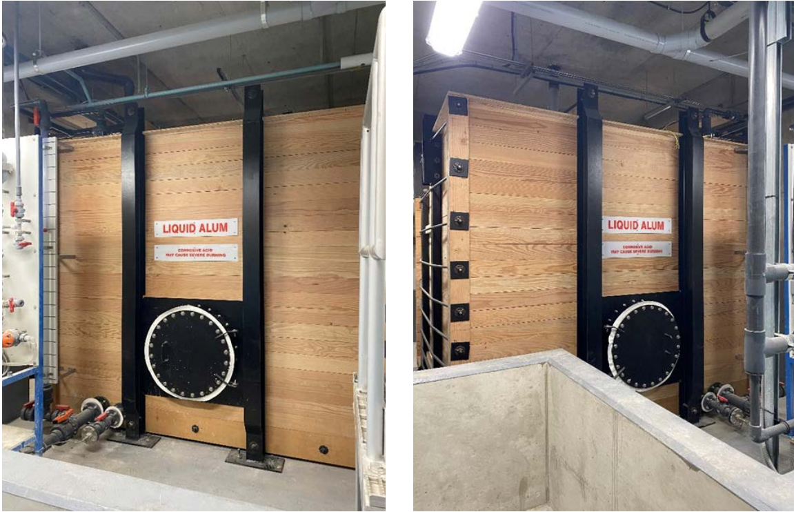
Figure 6a & 6b: New wood stave chemical storage tanks within a concrete secondary containment wall.
