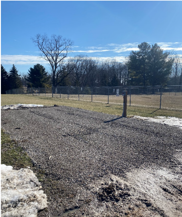
Figure 7: Gravel contractor trailer pad with a permanent electrical pedestal
