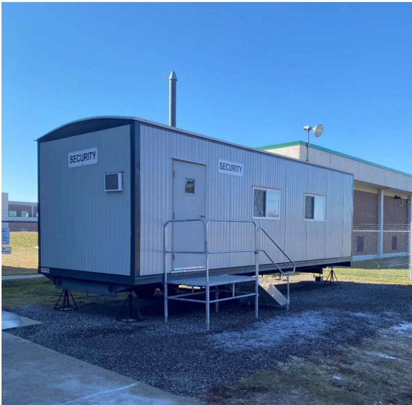
Figure 4: The new security trailer at the Elgin WTP.
