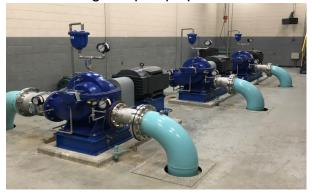
Thomas pumps are equipped with variable frequency drives (VFD) with each pump having a rated capacity of 263 L/s. With the current VFDs being utilized as soft and stop variable frequency drives.
