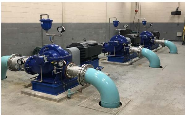
The St. Thomas pump station has two duty pumps and one standby pump. All three pumps are equipped with Variable Frequency Drives (VFD). However, the VFD's are presently configured to act as soft starts. Each pump has a rated capacity of 263 L/s.
