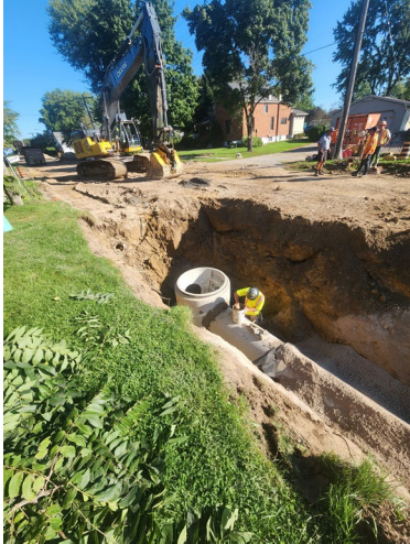
Storm Sewer Installation
