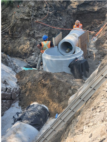
Storm Sewer Installation
