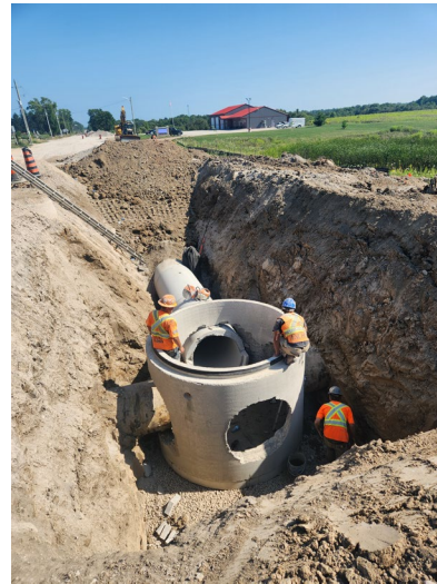
Storm Sewer Installation
