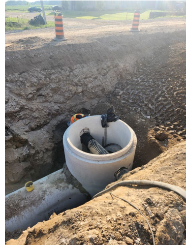
Storm Sewer Installation
