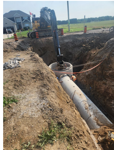
Storm Sewer Installation
