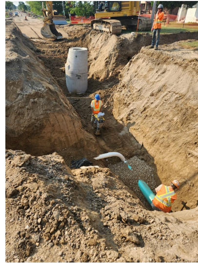
Sanitary Sewer Installation
