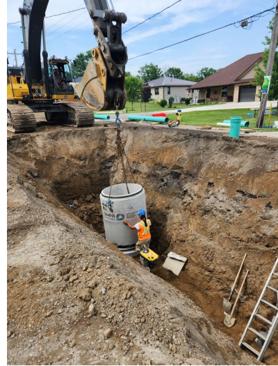
Sanitary Sewer Installation
