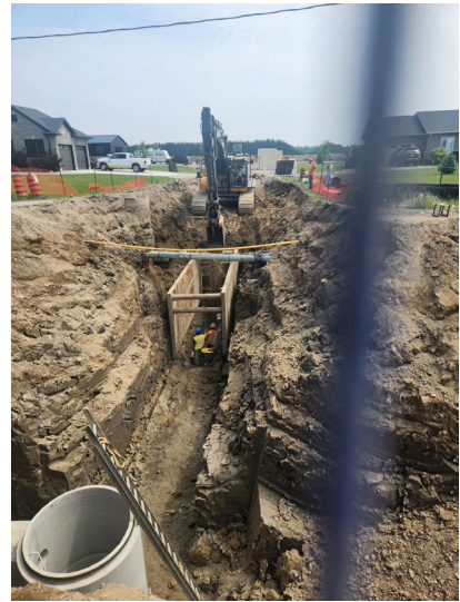
Sanitary Sewer Installation
