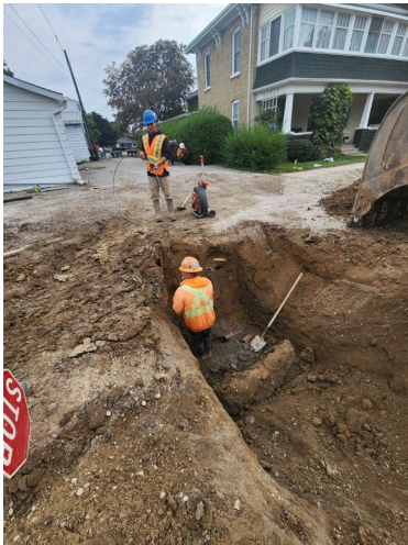
Storm Sewer Installation
