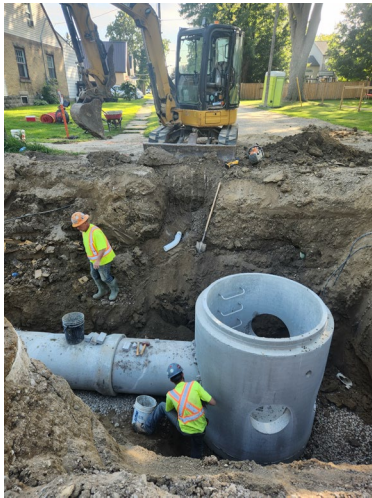
Storm Sewer Installation
